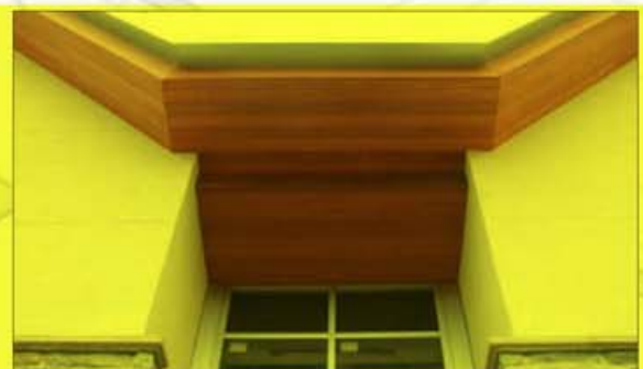
Millwork Chestnut Hill Academy Blasz Construction, LLC
