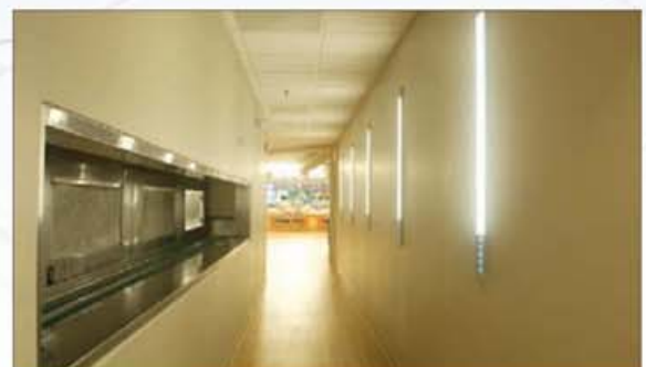
Drywall Finishing Johnson-Hardwick Dining Hall Sloan & Company
